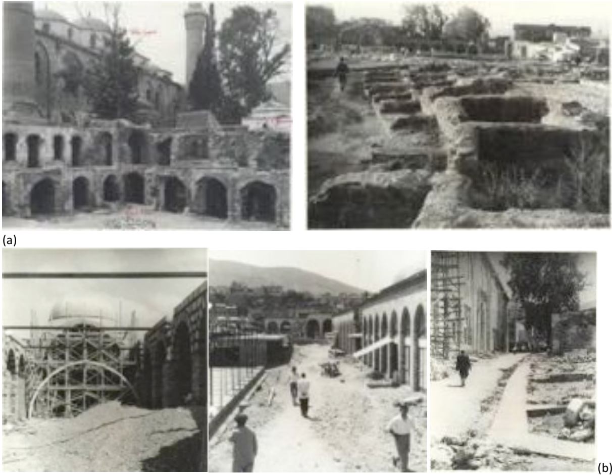
Figure 6. (a) Deformations in the monumental buildings of Hanlar Districts, photographed after 1958 fire, (b) Reconstruction and renovation applications by using reinforced concrete after 1958 fire (source: archive of Umut Ünsal, from the archive of Bursa Metropolitan Municipality (BBB))
